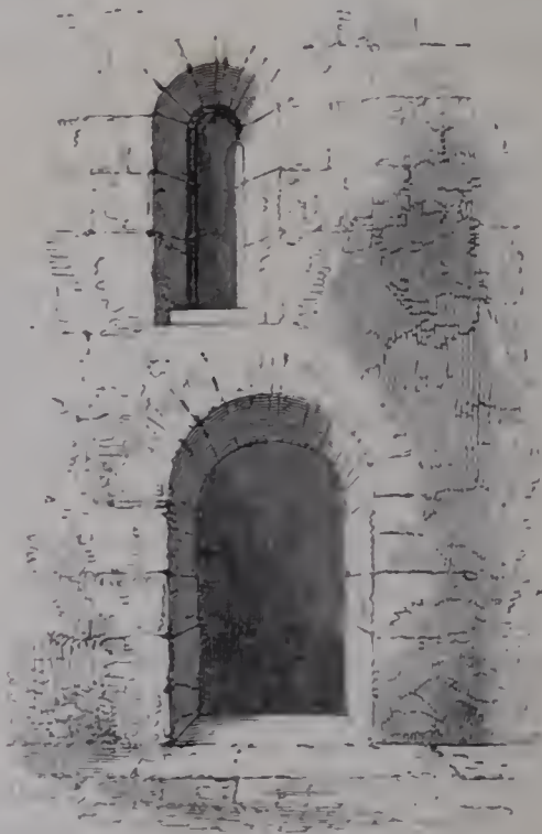
Anglo-Saxon Doorway and Window, interior of the tower of Brigstock Church, side.
